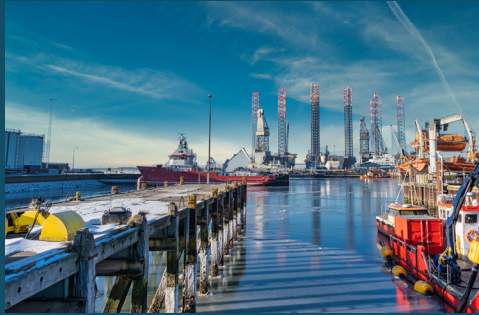
600kW onshore power at the Port of Esbjerg
