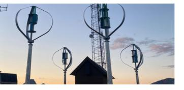
Ballard has collaborated with Eltek on the <u>project Trollstigen</u> in the mountains of Norway, installing an off-grid power solution that integrates solar, wind, fuel cells from Ballard, and batteries to ensure continuous operation and connectivity of a remote telecom network site. The fuel cells provide backup power to the site, when no alternative sources are available and ensures constant connectivity.
